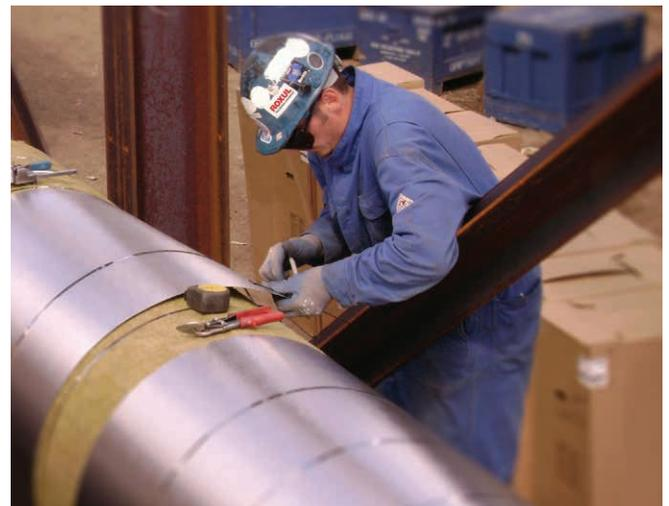
ProRox PS 960<sup>NA</sup> requires nothing more than a serrated knife for precise cuts that can be made quickly and easily at the point of installation, reducing waste and manpower hours.
