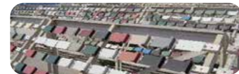
Bellambi Point site, Australia
