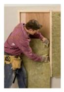
To install simply push in the specially designed flexible edge.
