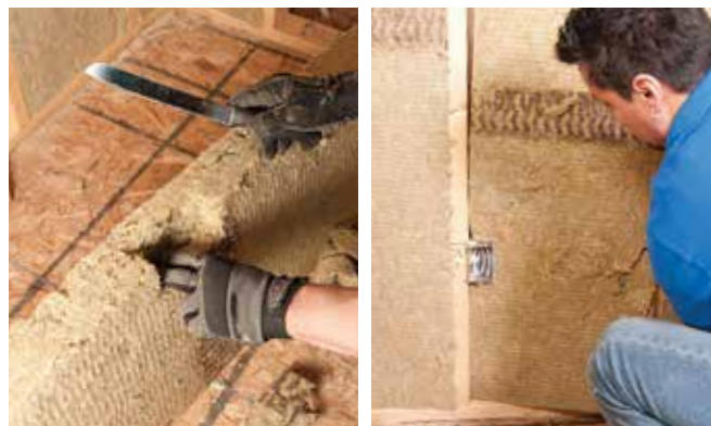
ROXUL COMFORTBATT® higher density batts make it simple for precise cutting to ensure a fit without gaps and voids.
